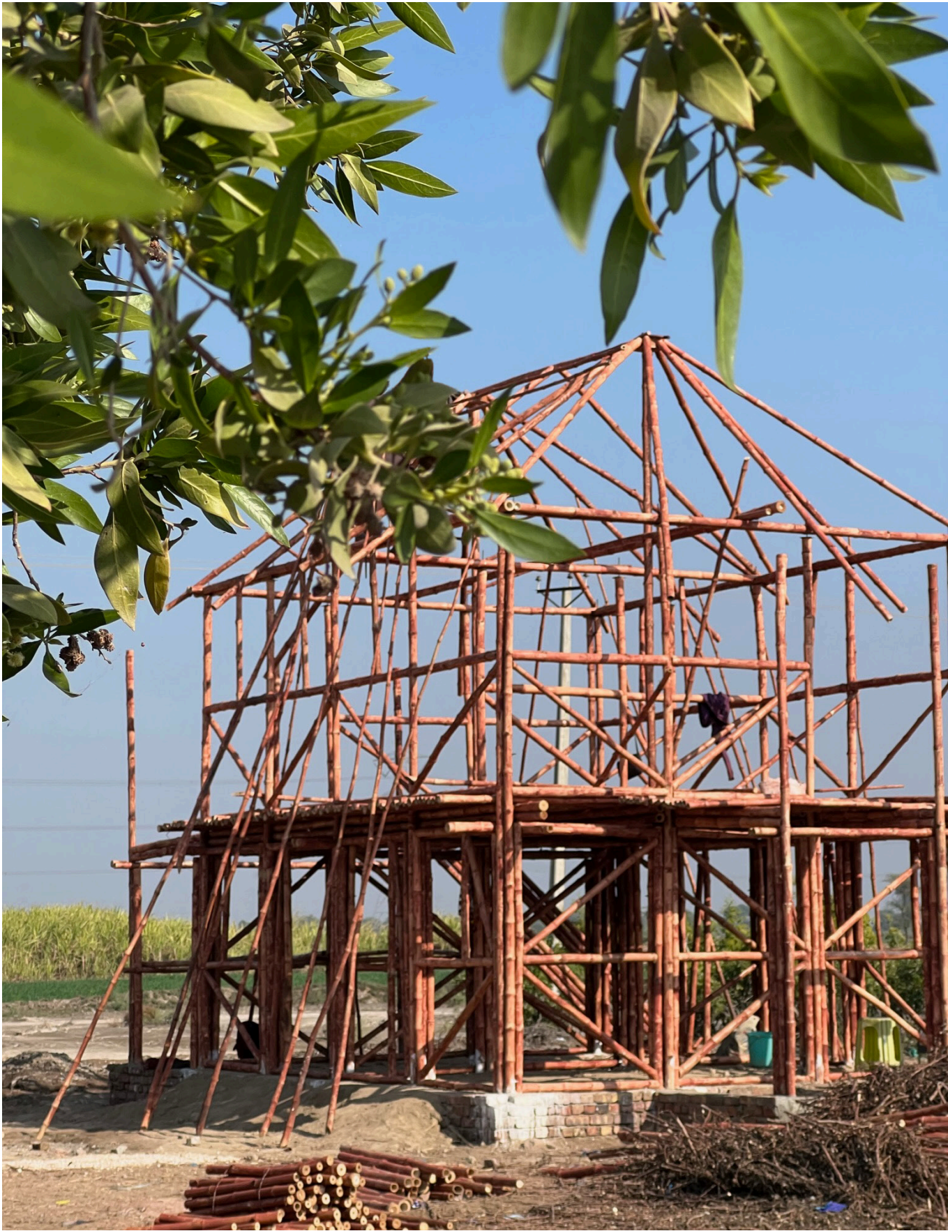
Nyami Noohani School under construction
